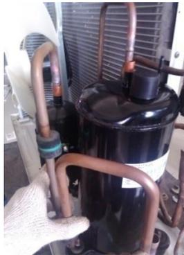
Defective Samsung Compressor, By De-brazing suction & Discharge Tube Take Out The Compressor Remove One Bolt As Shown, Keeping Two Bolt In tag, Place the Adapter plate In Basepan As Shown
